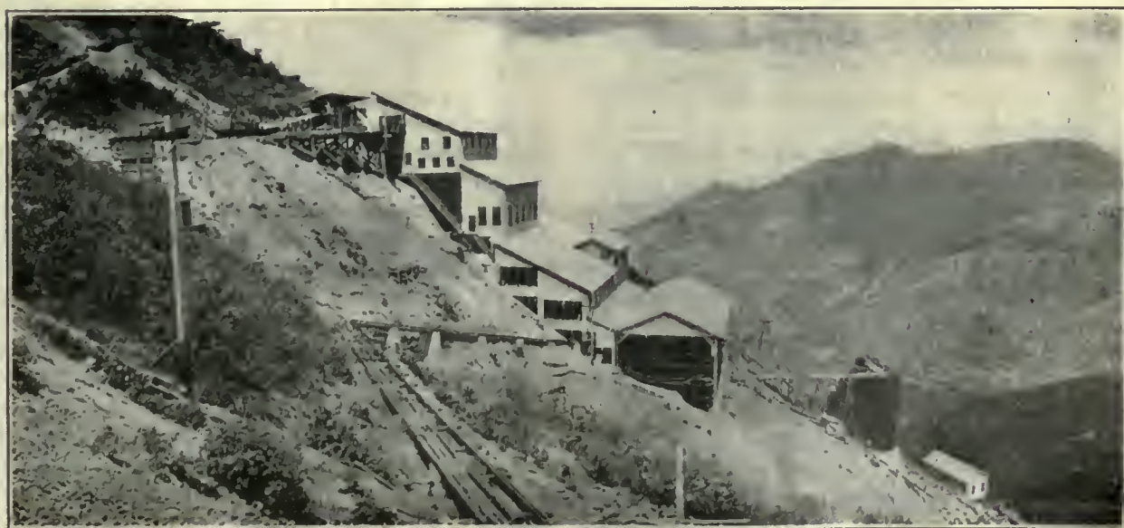
FIG. 2. GENERAL VIEW OF MILL.
